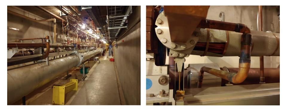
Large pipe is laser tube with Fresnel Lens for alignment as a strong back. Accelerator runs very warm for temperature stability
